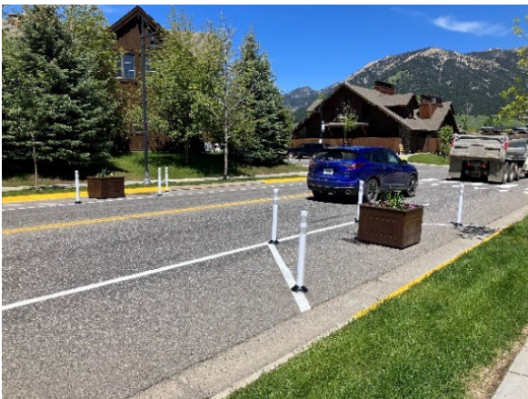
Figure 25: Pop-up curb extensions in Big Sky, MT (Photo: WTI)
