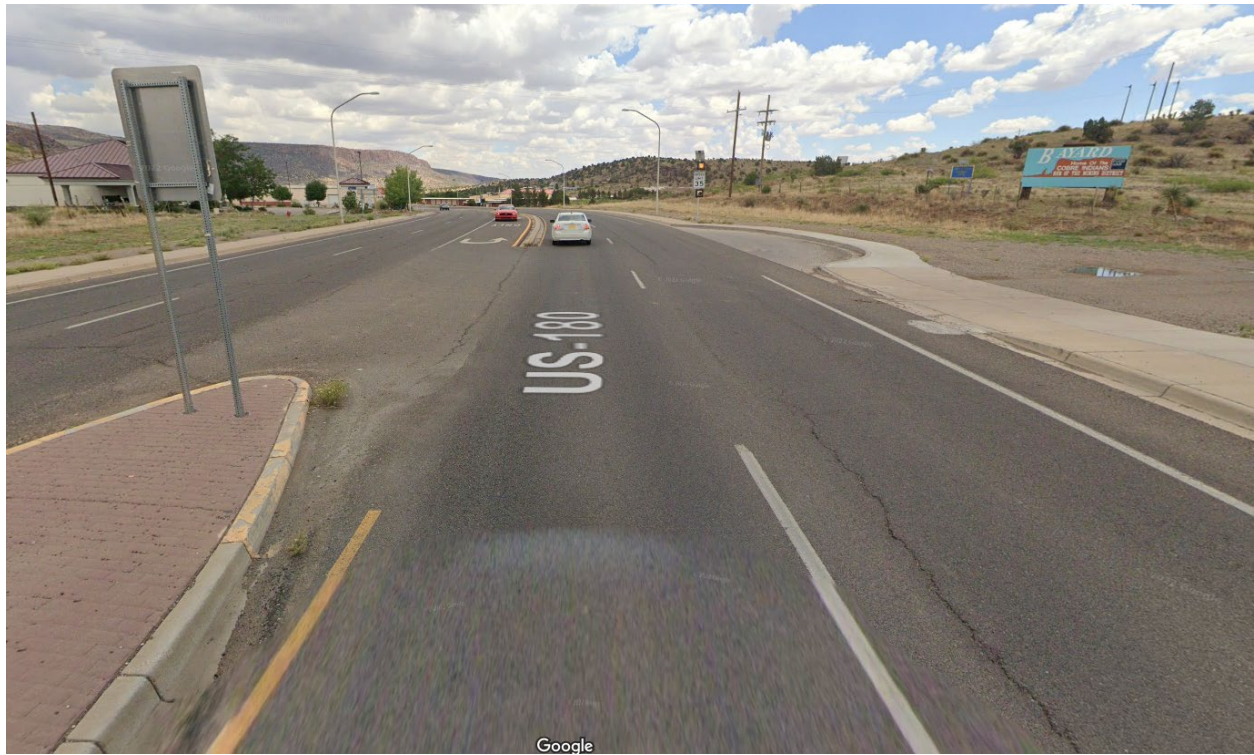
Figure 64. U.S. 180 East at Bayard Municipal Limit – Corridor Section 4 (Google, n.d.)
