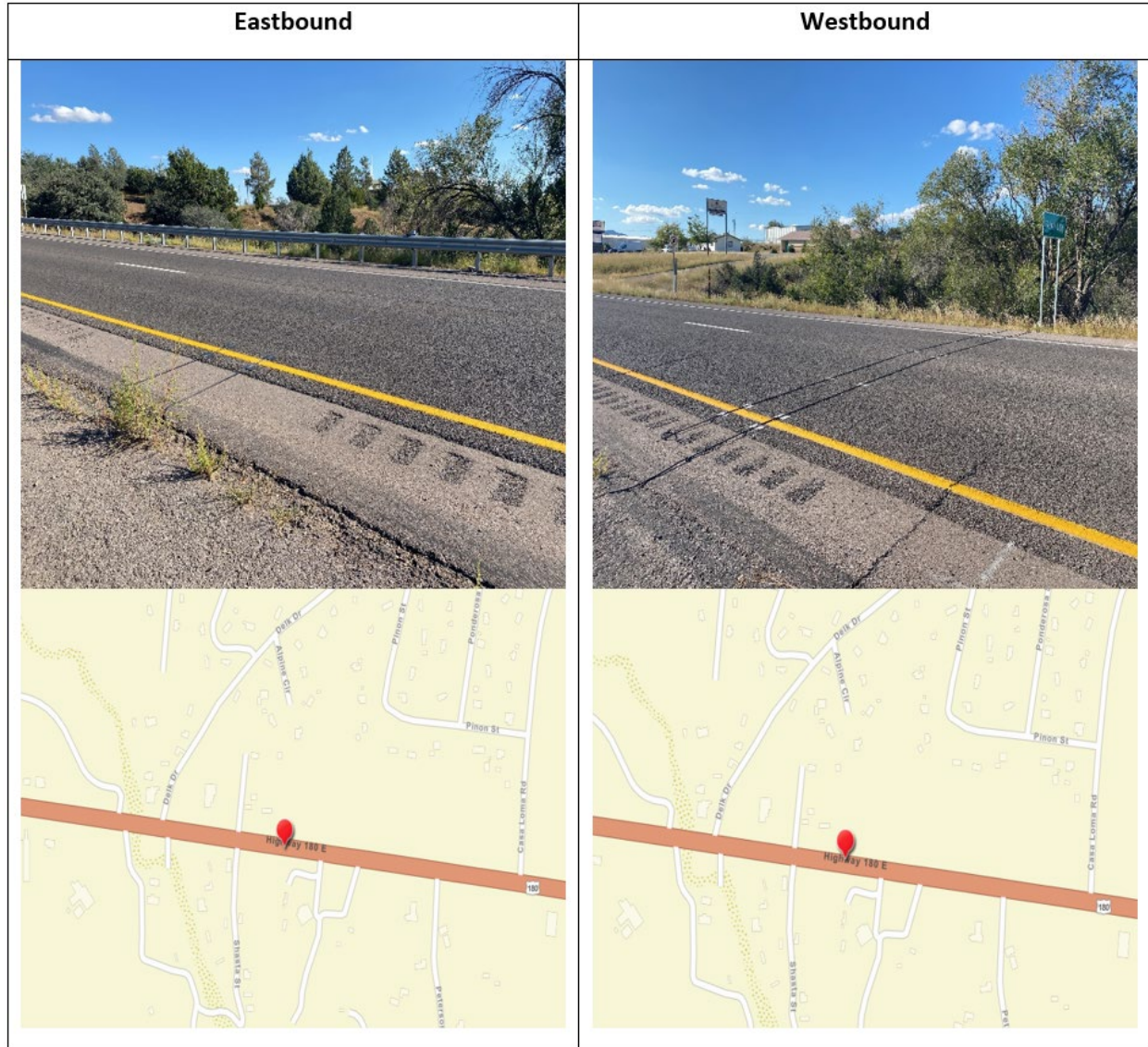
Figure 19. JAMAR Counters, Near E. Shasta Road (Esri, HERE, Garmin, FAO, NOAA, USGS, OpenStreetMap contributors, and the GIS User Community, 2023)
