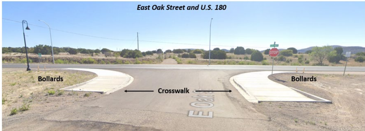
Figure 79. Crossing of East Oak Street
