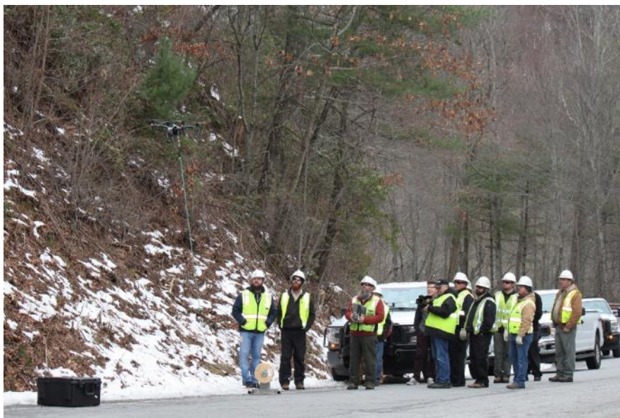
A drone pulls a broadband cable to connect infrastructure at Neels Gap, GA.
