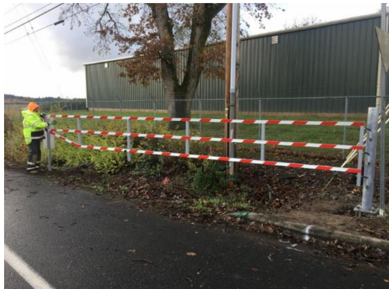
A Washington County Operations employee opens an arm of the Fern Hill flood gate.
